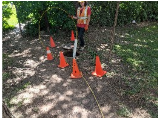
4. 30 Speers Road, MH SAN-2 (Likely buried MH STM-2-BURIED)
