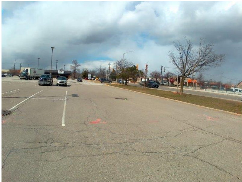
Photo 6 - View of associated parking lot area on Site, west of the on-Site buildings (facing north).
