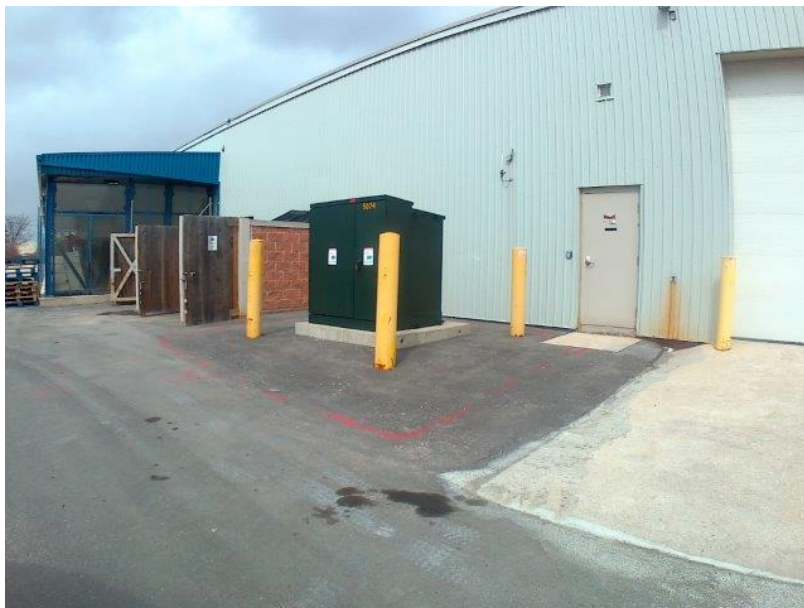
Photo 2 – View of the rear of the On-Site building (facing northwest)
