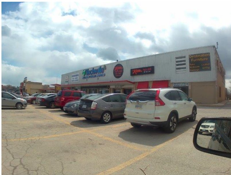
Photo 4 - View of front of the neighbouring property to the north (facing southwest).
