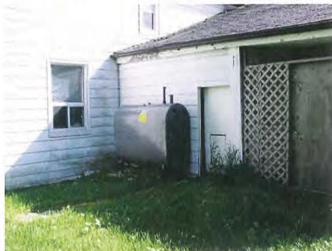
Offsite fuel oil tank in good condition.
