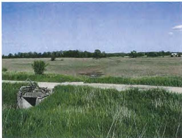
Offsite concrete culvert directing storm water southeastward flow onsite
