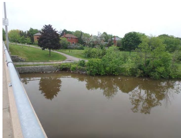
Photo 4: C2 northwest bank.
