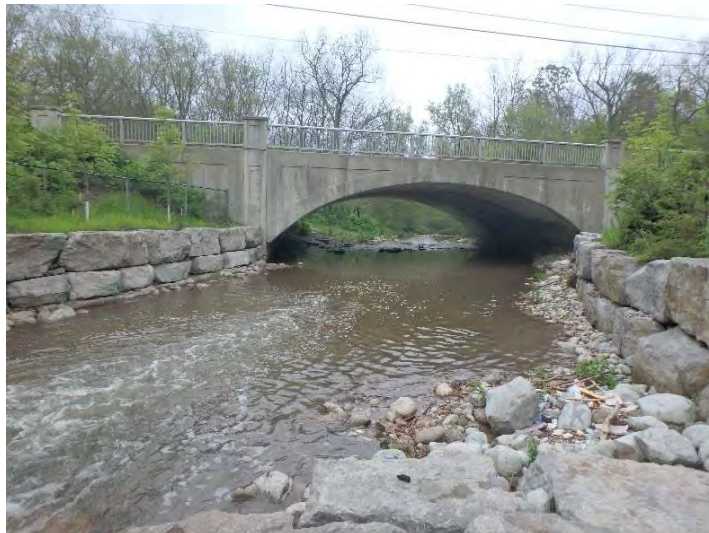
Photo 31: Crossing C11 facing south.
