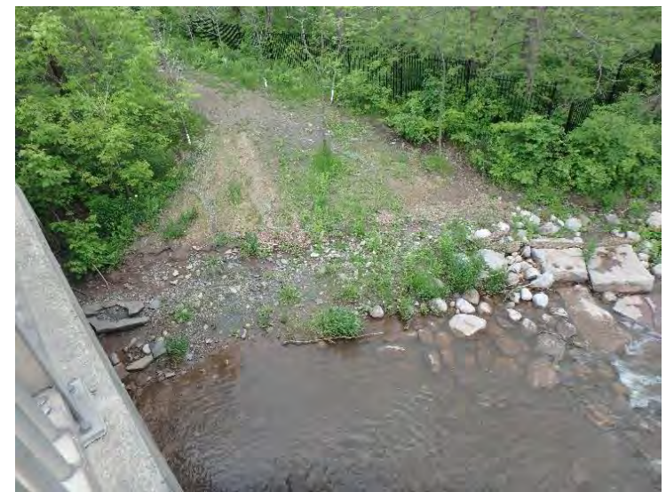
Photo 36: C11 southeast bank of bridge.
