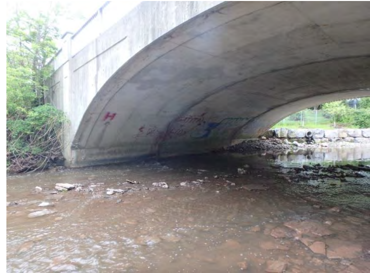
Photo 34: C11 east side of bridge.
