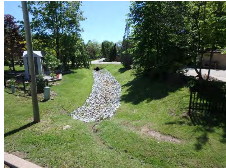
Photo 52: C18 downstream of Lakeshore Road ROW.
