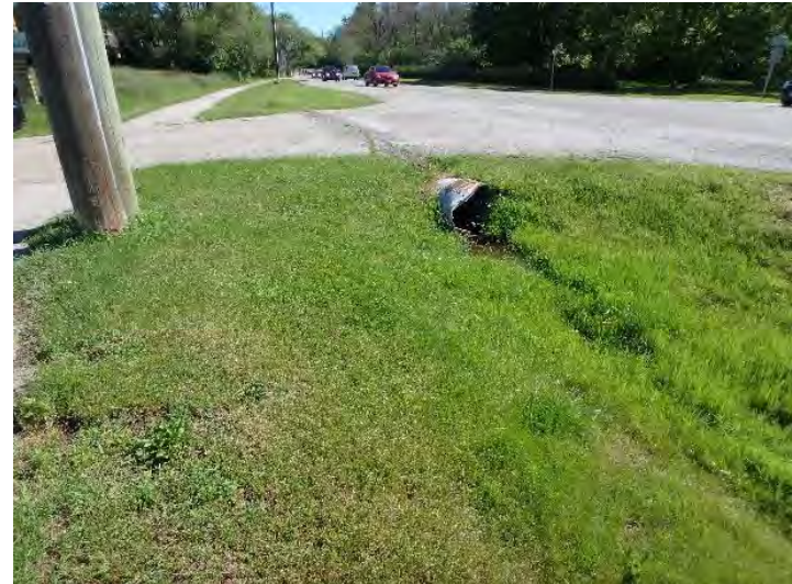
Photo 30: Crossing C10 west side.
