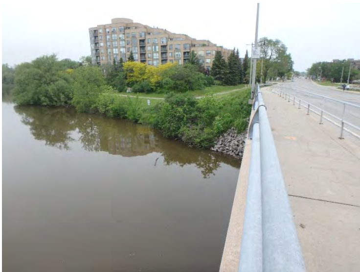
Photo 5: C2 northeast bank.
