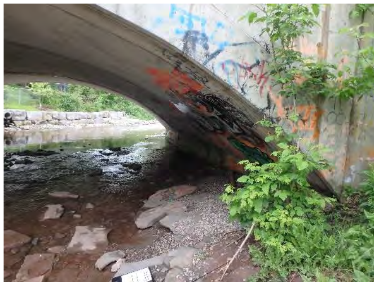
Photo 35: C11 west side of bridge.
