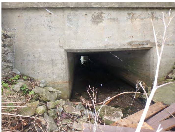
Photo 27: Bridge at C8.
