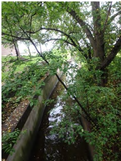
Photo 25: Crossing C8 downstream of ROW.
