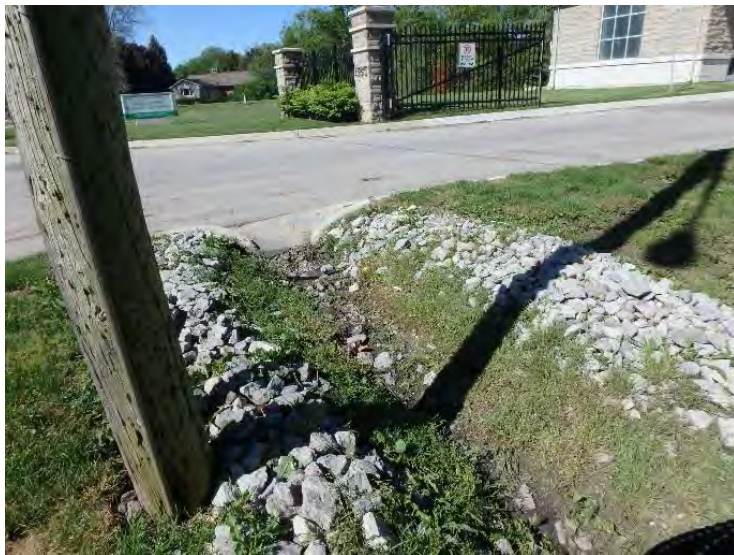
Photo 23: Crossing C7 facing west.
