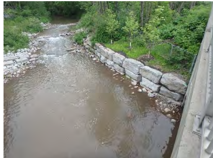
Photo 32: Crossing C11 northeast bank.
