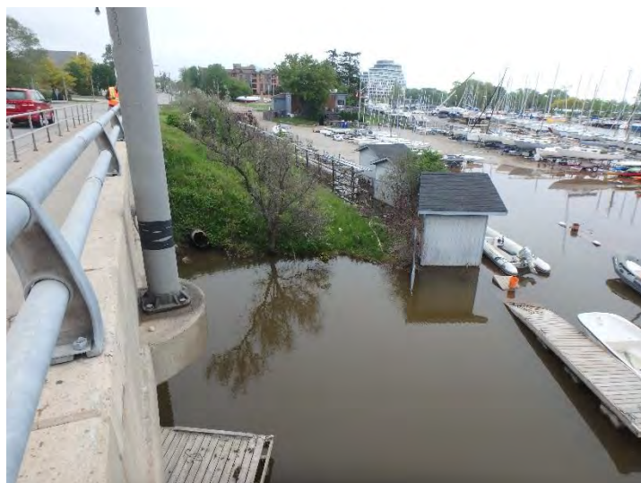
Photo 7: C2 facing southeast bank.
