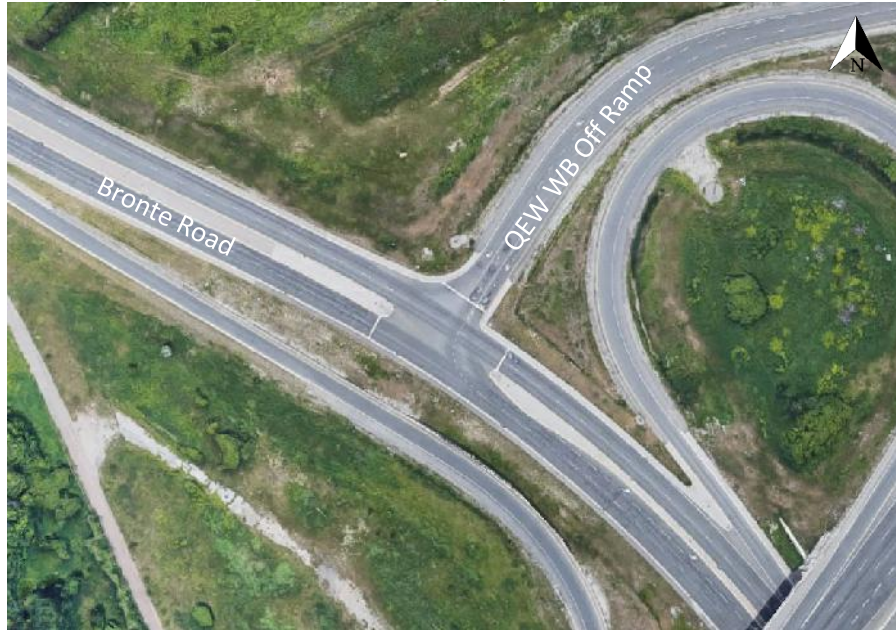
Figure 6: QEW WB Off Ramp at Bronte Road
