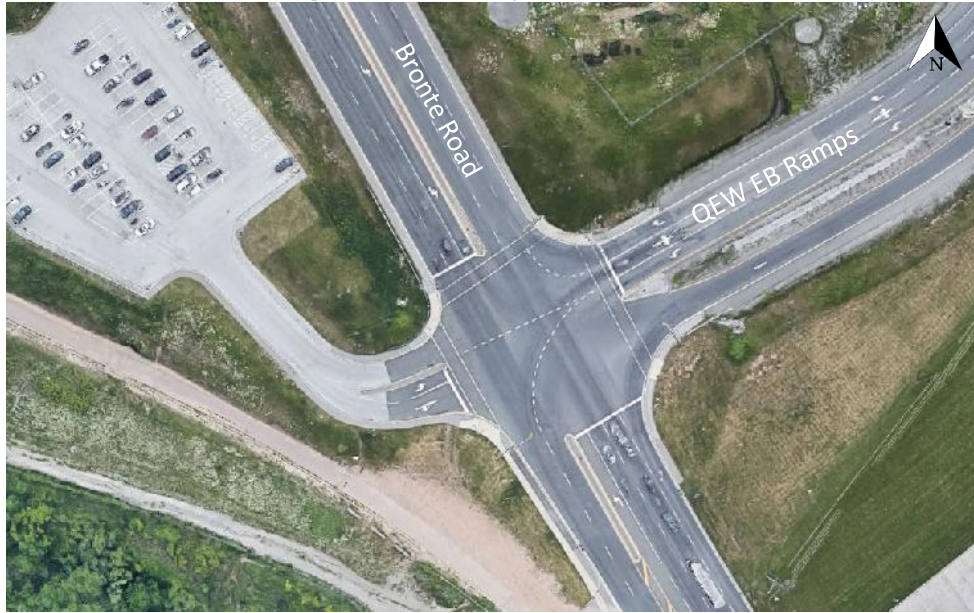
Figure 7: QEW EB Ramps at Bronte Road
