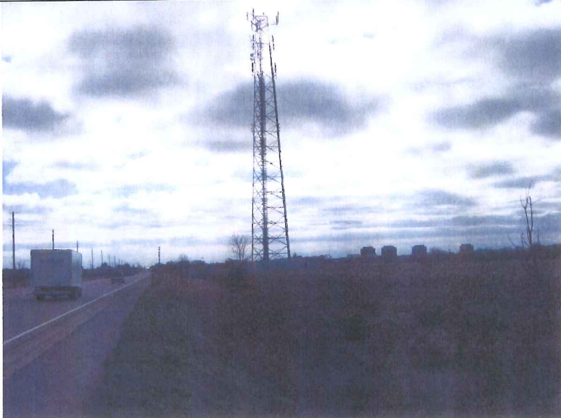
Transmission tower on the northeast adjacent property
