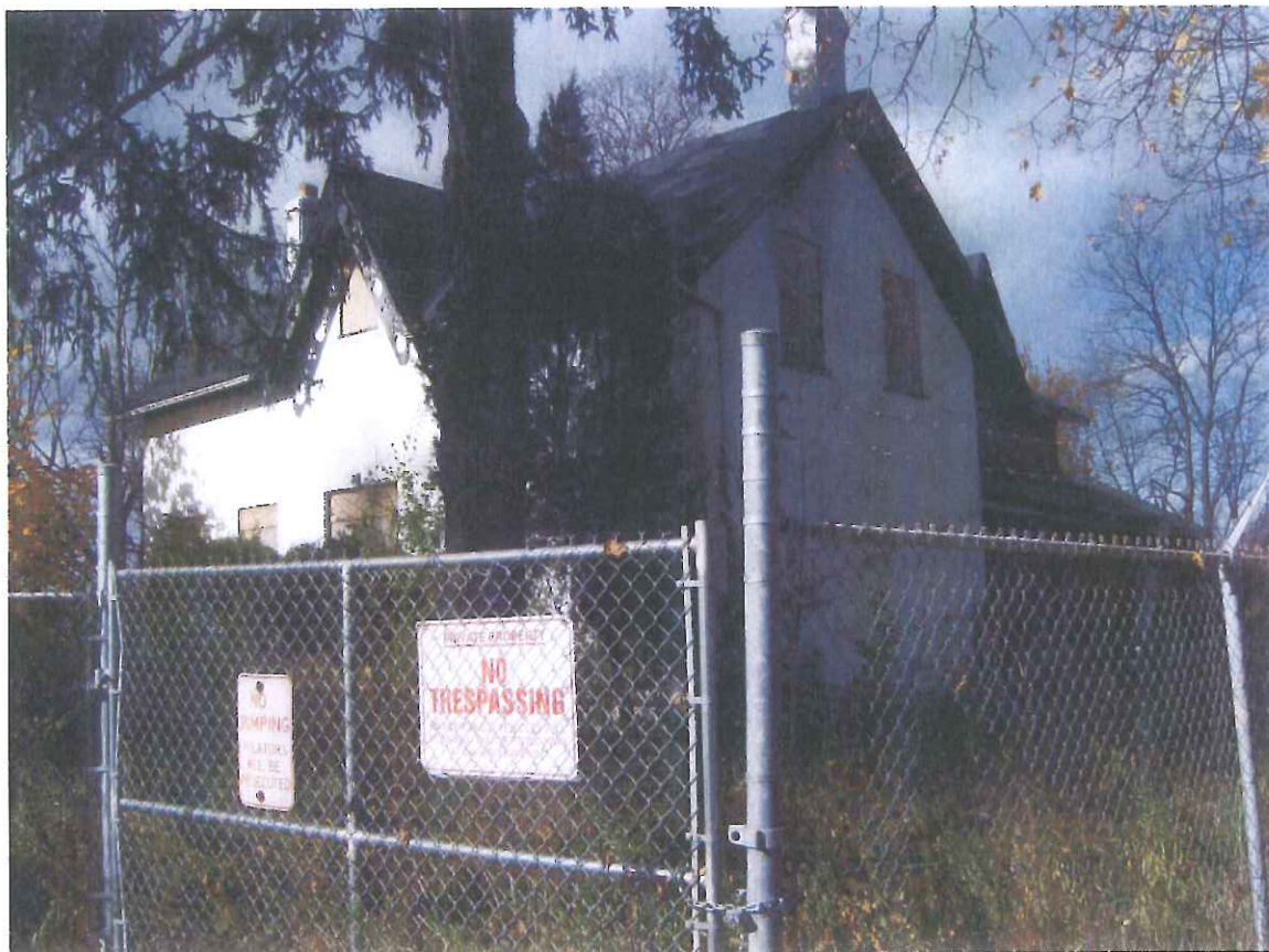
Abandoned house at 257 Dundas Street East
