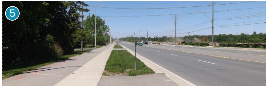
View facing north on the west side of Bronte Road
