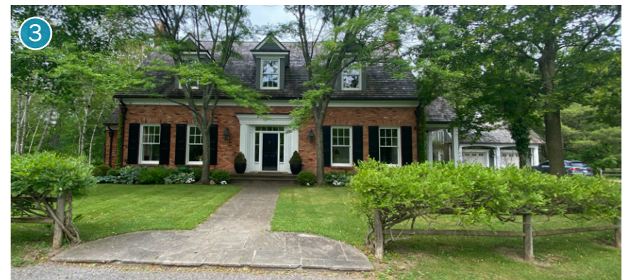
Front exterior view of the existing Enns House
