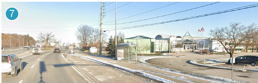
View facing north from Bronte Road of Halton Regional Centre
