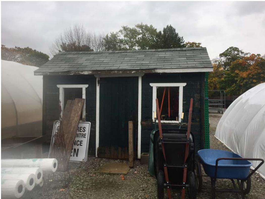
General view of a shed located at the Phase One Property (facing east)
