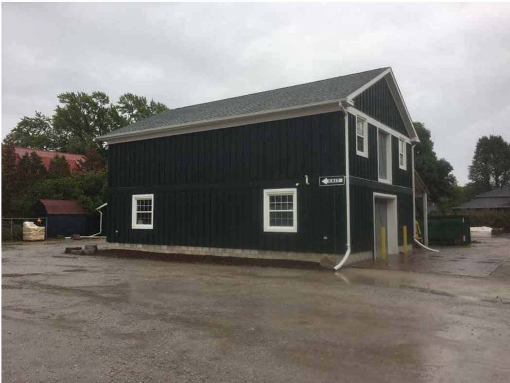
General view of the barn located on the Phase One Property (facing south)
