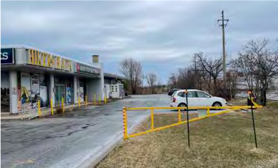
2 Subject Site, Vehicular Entrance
